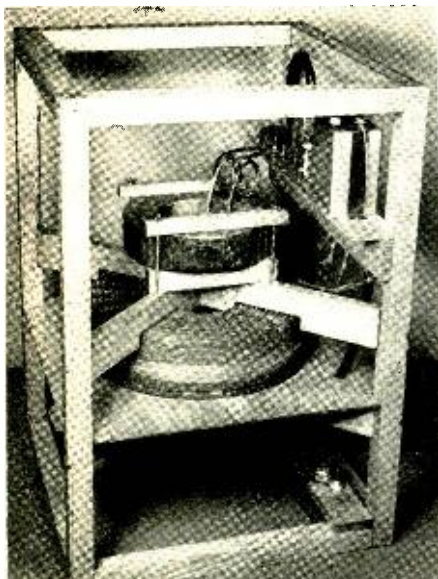
Fig. 4. Two-frequency wave trap.
